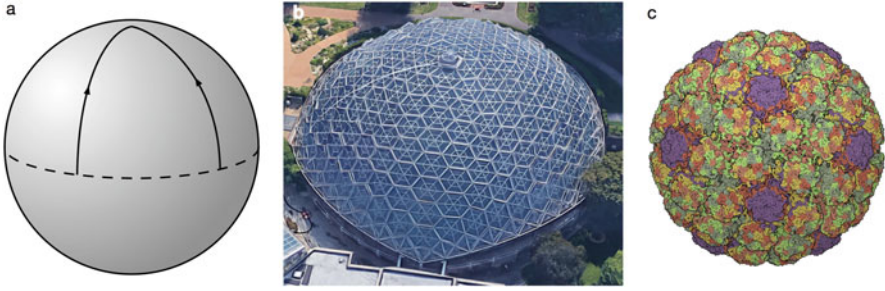
Fig. 1.4 Gaussian curvature constrains geodesic curves, tilings of space, and the existence of defects. (a) Two paths emanating north from the equator converge due to the positive Gaussian curvature of the sphere. (b) The Climatron in St. Louis, Missouri is a geodesic dome with a single, pentagonal disclination as its capstone and five kinks along its boundary. Topologically equivalent to a disk ( \chi = 1 ), the dome compensates for the integrated Gaussian curvature via the disclination and the discontinuities along its boundary. Image courtesy of Google Maps (Imagery ©2018 Google, Map data ©Google) [20]. (c) The human papillomavirus (HPV) uses 12 pentagons to form a spherical viral capsid. Qutemol image of 1LOT courtesy of Dr. J.-Y. Sgro, UW-Madison (©2009 Jean-Yves Sgro) [21]
